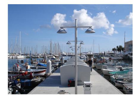
Moorage at Cannes Commercial Fishing Docks were significantly improved thanks to a complete upgrade to the Port's floating piers. Bellingham Marine led the renovation which included the replacement of the marina's existing pontoons with modern concrete floating pontoons Unifloat® anchored on pilots as well as upgrades to the marina's power, illumination and potable water systems.
